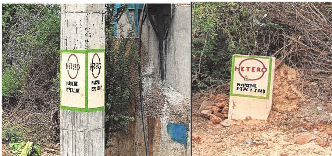
Permanent Display Boards installed at Road & Creek crossing along pipeline
