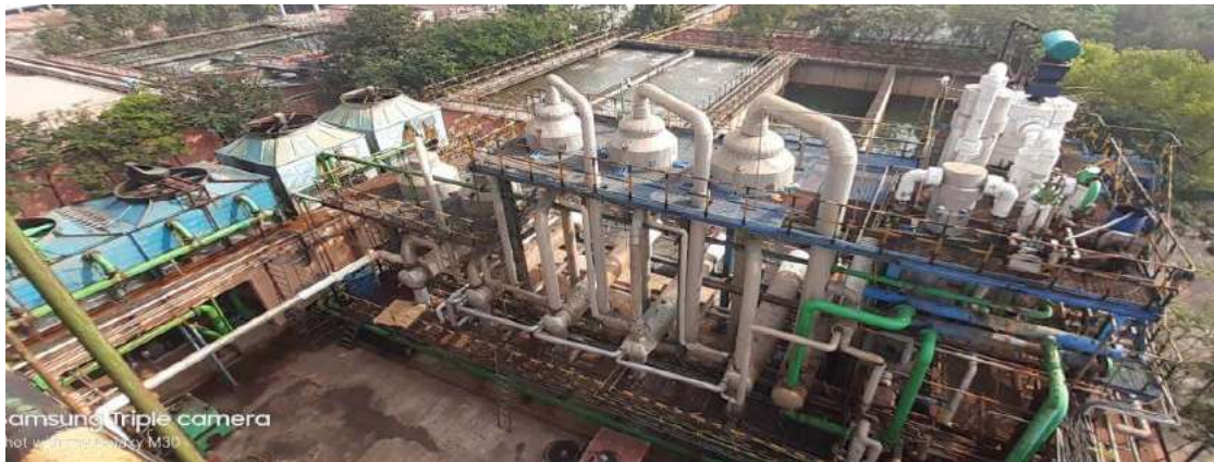
Multiple effect evaporator
